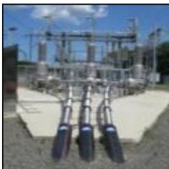
**Superconducting Cables** Superconducting technology is considered a new means to increase the capacity and reliability of electric suppliers' systems. It can carry three to five times more power than conventional cables. Nexans designed and manufactured the cable, and its cryogenic envelope, for the world's longest and most powerful superconductor cable to date - integrated into a live transmission grid for the Long Island Power Authority in the US.
