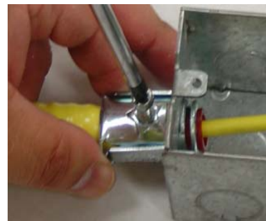
Figure 2 Interlock Armor Bonded. Optical Cable Core Continues
