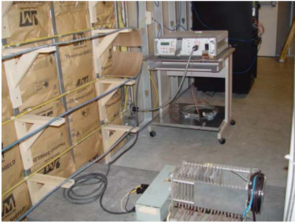
Figure 3: Haefley Generator and heat sink.
