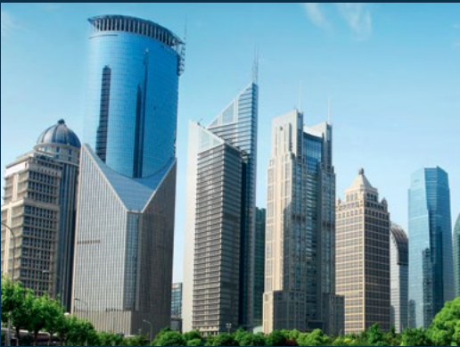
Building & Territories (including utilities & emobility)
